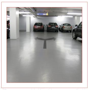
ACRYLICON VARIANT SYSTEM IS A MONO-COLOUR SELF LEVELLING SYSTEM. IT CAN BE LAID IN VARIOUS THICKNESS FROM 1MM TO 3MM DEPENDING ON THE LEVEL OF IMPACT RESISTANCE REQUIRED. WITH A 98 N/MM2 COMPRESSIVE STRENGTH, ACRYLICON VARIANT SYSTEM IS ULTRA-CLEANABLE. SLIP RESISTANCE CAN BE ALTERED TO SUIT EXACT REQUIREMENTS.
